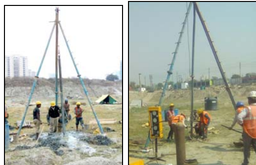
Fig. 8. Boreholes and pressuremeter tests in progress
