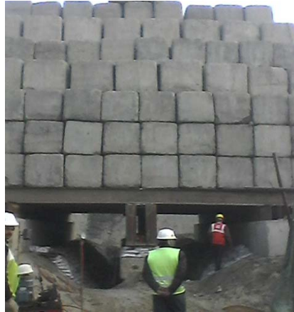
Fig. 6. Pile load test in progress
